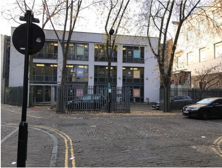
Image 3: View towards the site from the east and Kingsland Passage
